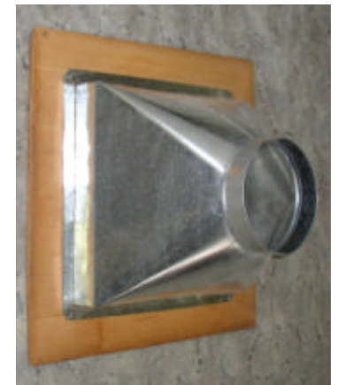
Register Boot w/ Flange attached to plywood
